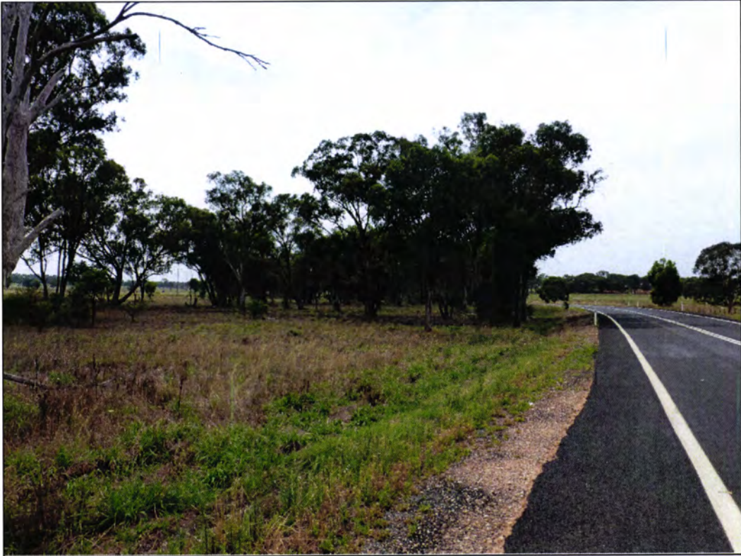
Plate 4: Looking west along the Castlereagh Highway with the rehabilitation reserve on the left
