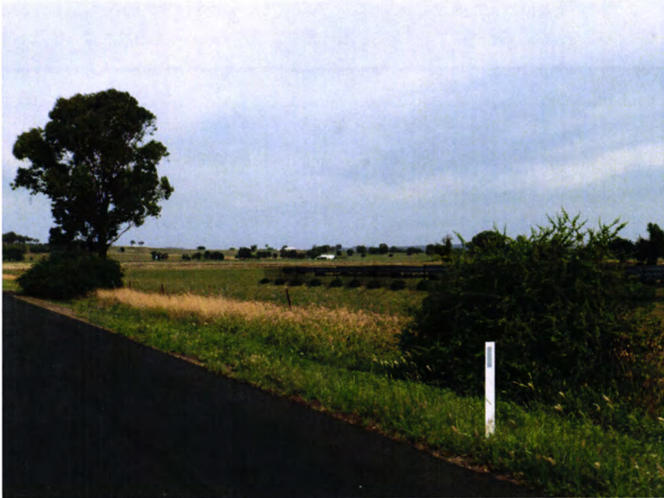
Plate 2: The solar farm and security fencing after initial screen planting
